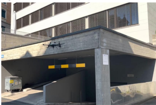
Figure 3: Drone horizontally tilted inspecting a building
