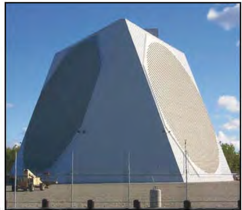
Like the eyes of a giant insect, the 90-foot diameter phased array radar scans the northern sky. Alaska District managed the $47 million Clear Radar Upgrade. (Photo courtesy of Alaska District)
